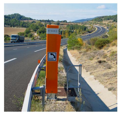
The architecture of the network is composed by optical bus **able to drive up to 50 couples of ECB (100 Emergency Call Boxes)**.
